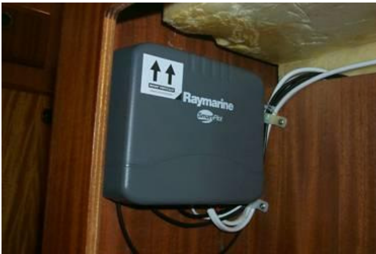
Installation of Flux Compass & Core Pack on Sea Dragon
