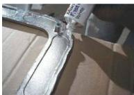
Once I felt the ports were well seated, I removed the screws & trim ring and filled in any gap in the butyl rubber caulk... Finally, following the NFM instructions applied a Boatlife polysulfide sealant. I know - some would suggest 5200... Not me see FRAME
