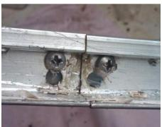
The fixed port is held together by four screws (2 on each side). The screws pass through the aluminum frame into an aluminum "backing plate". Once the screws have be removed the frame can be split into two (2) pieces and the glass and gasket removed.
